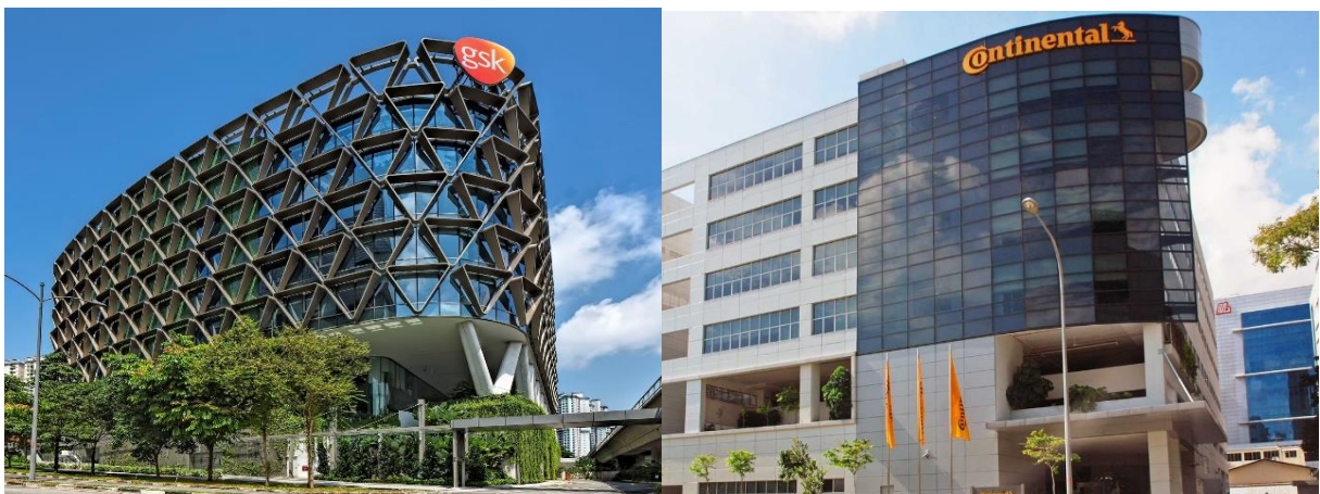
From Left to Right: GSK Asia House, Continental Building – Phase 2
